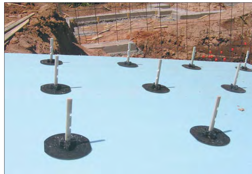
A close-up of the rigid form insulation and unique tie system used to suspend the insulation between the forms.
